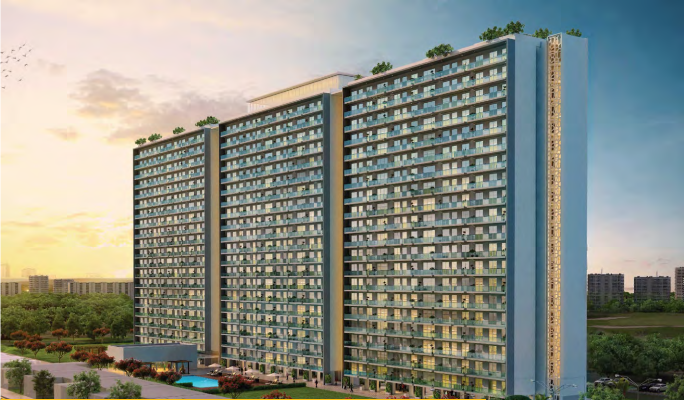
22 Storey - Godrej Golf Link Project, Cluster B Towers - India
