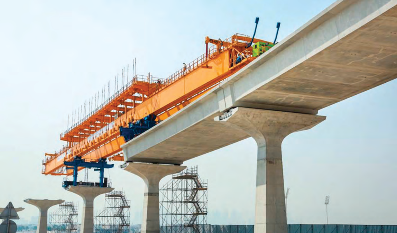
QATAR RAIL RED LINE ELEVATED PROJECT
