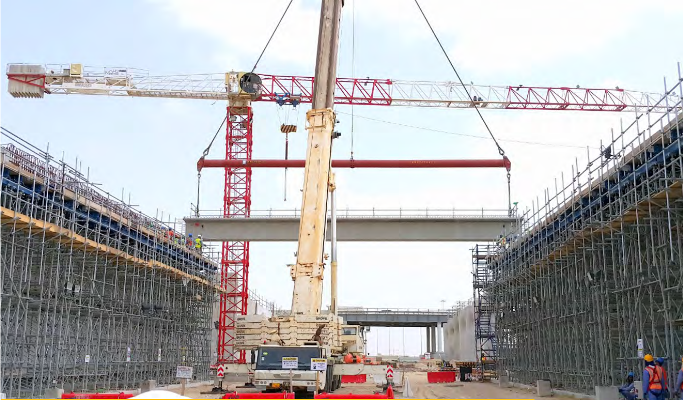
ERECTION OF GIRDERS AT AL KHOR HIGHWAY PROJECT
