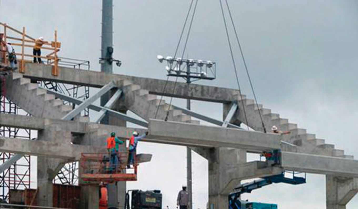
PRECAST RACKER BEAMS
