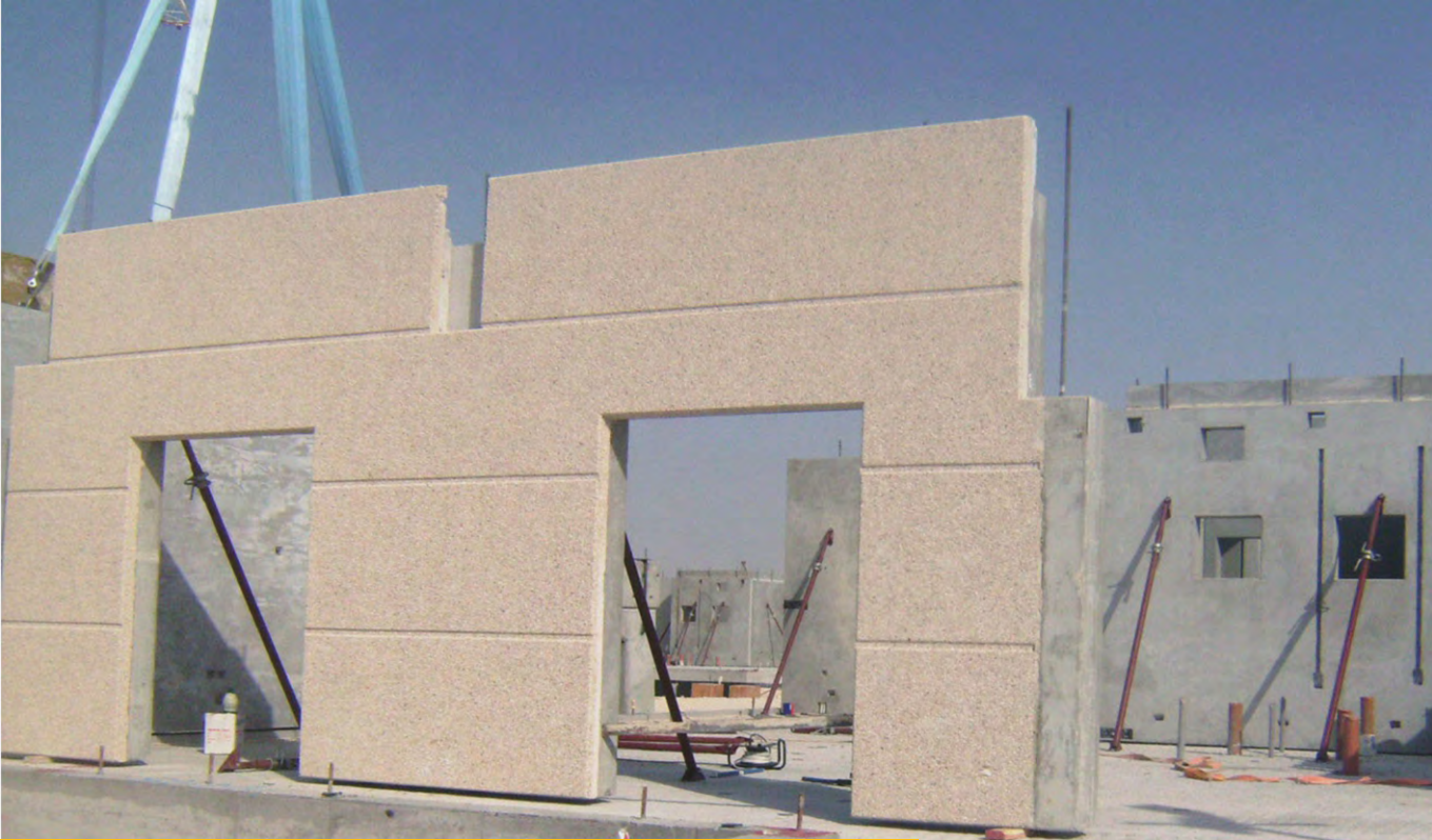
PRECAST INSULATED WALLS AND CORE WALL
