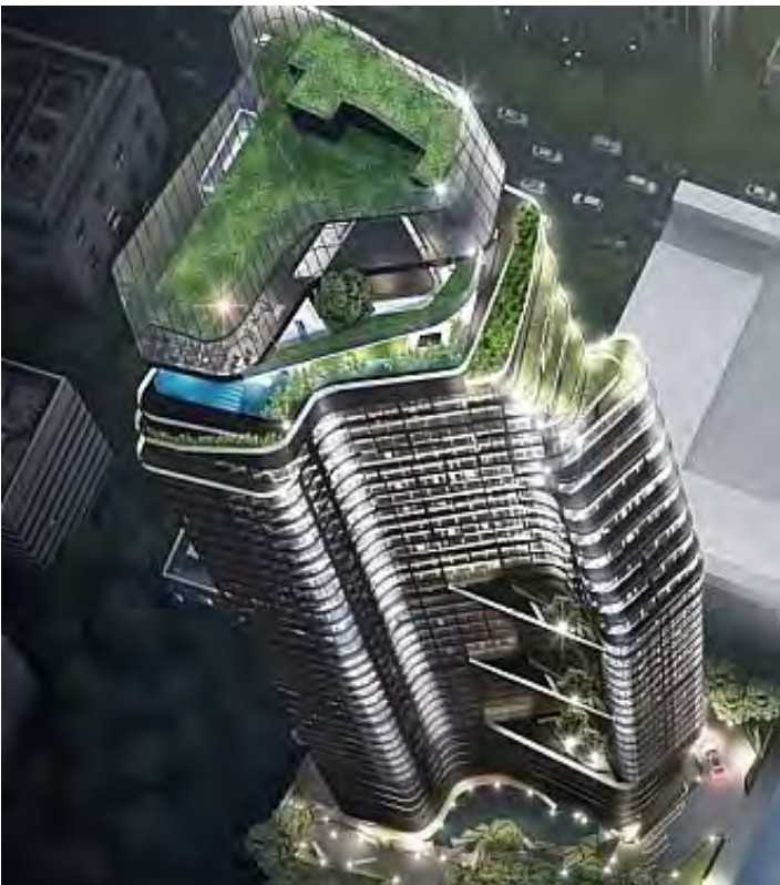
39 Storey - Ideo Q Victory – Residential tower – Thailand
